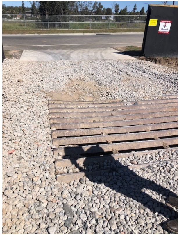
Photos 1 & 2: Heavy vehicle wheel wash and cattle grid at site exits to Conferta Avenue
