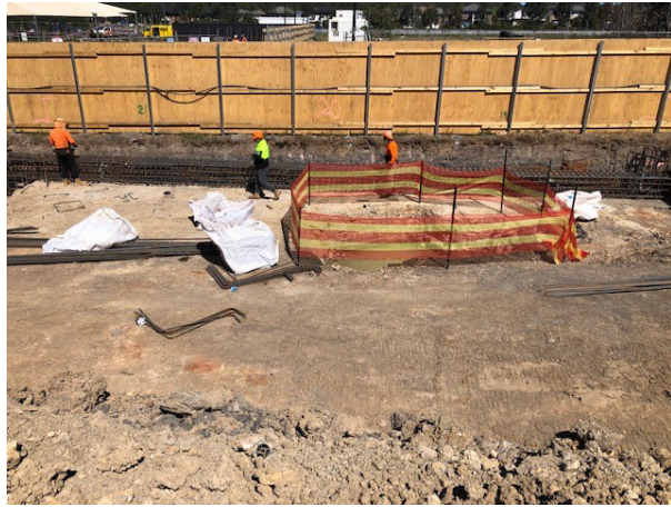
Photos 9 & 10: Accumulated rainwater in low excavation and piles. Deicorp advised no dewatering had been conducted to date.
