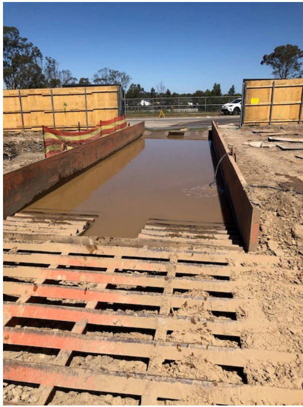
Photos 1 & 2: Heavy vehicle wheel wash and cattle grid at site exits to Conferta Avenue
