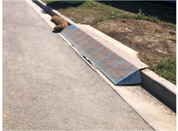
Photos 3 & 4: Covered load of spoil and drain controls on Conferta Avenue
