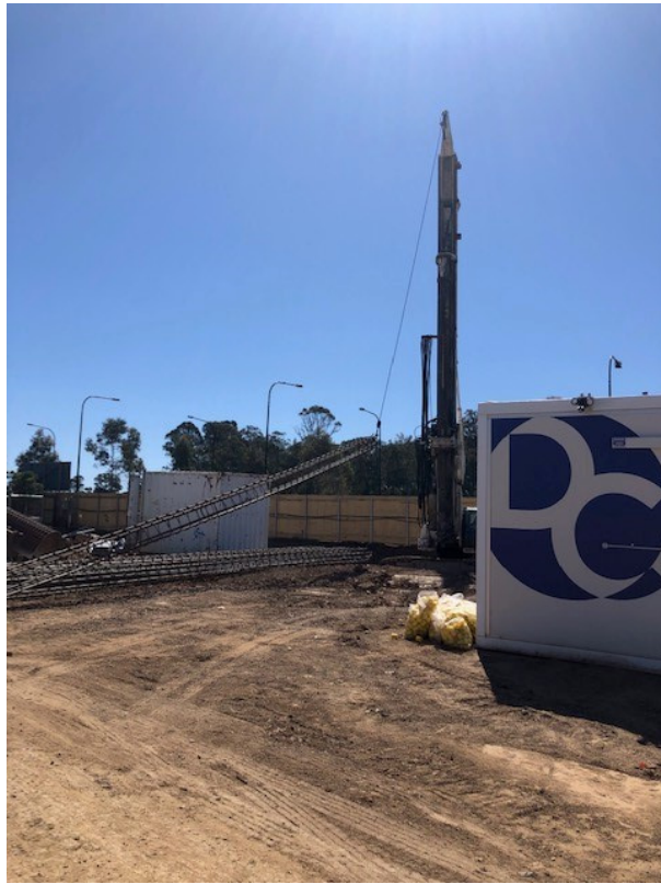
Photos 5 & 6: Drill piling along the norther site boundary
