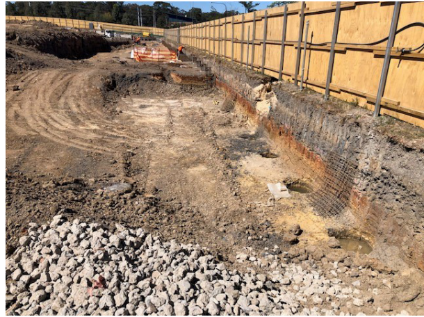
Photos 9 & 10: Accumulated rainwater in low excavation and piles. Deicorp advised no dewatering had been conducted to date.
